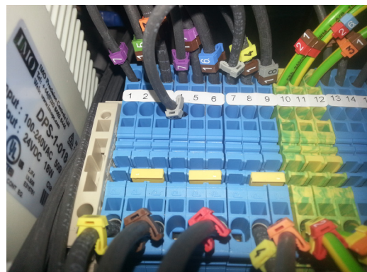
Delta Configuration: Jumpers across 2-3; 5-6; 8-9
